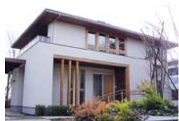
The Universal Design House, which can be stayed in overnight, is used for real-time, actual design verification and employee training. It also incorporates Ryouonbou design.
