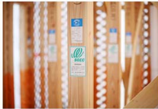
All standard studs feature the SGEC certification symbol, demonstrating the use of certified timber
