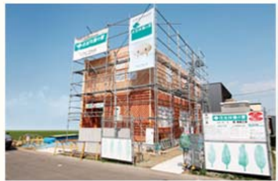
The residence under construction
