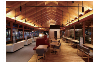
Example of wood construction (restaurant)
