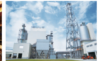
Mombetsu Biomass Power Plant
