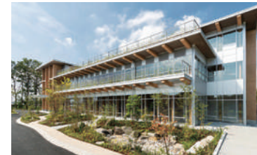
New research building at Tsukuba Research Institute
