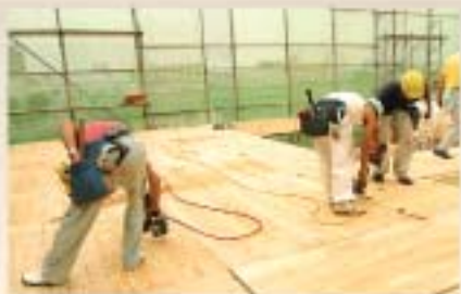
The "Durable Floor Panel" plays a crucial role in dispersing the lateral shaking force of earthquakes without exerting a load on individual walls
