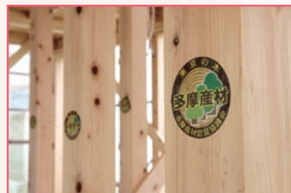
Timber from the surrounding mountains is used in the homes' principal structural members
