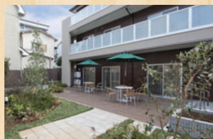
A wooden private elderly-care facility (two-by-four system, three stories)
