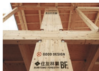
Large columns (engineered wood) used in the BF construction method
