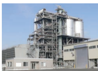
Wood-chip biomass power plant (Kawasaki Biomass Power Plant)
